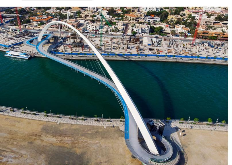
lifted then on the top of temporary towers, reaching at their tallest point 53 meters of height, by means of two 600-tons crawler cranes. The weight of the arch alone is 1.700 tons and, through 20 steel cables (for a total length of 858 meters), supports the S-shaped deck, 6.7 meters wide,
